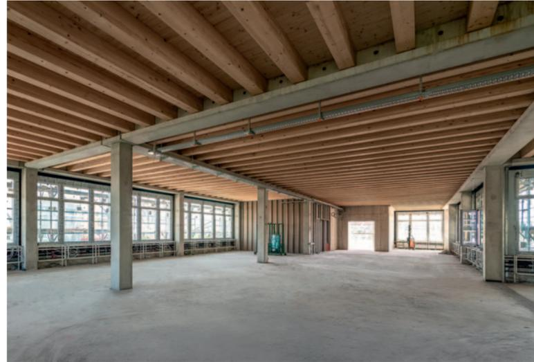
Die Holz-Beton-Hybriddecken made by Dreßler Bau
